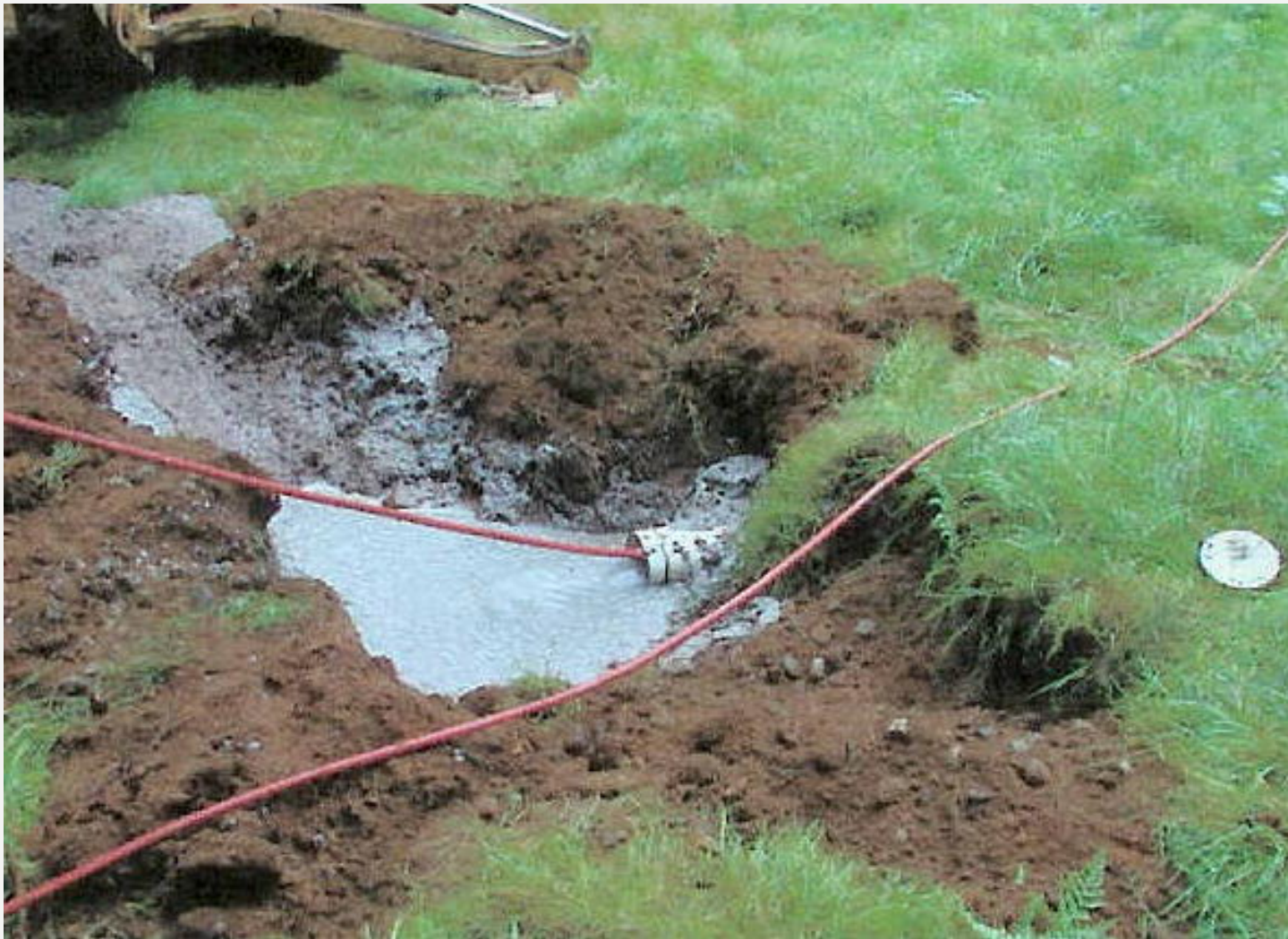
Removing Contaminated Sludge
